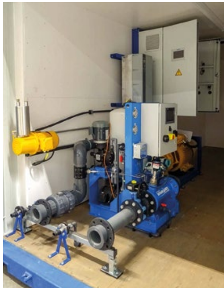
The Uniballast system fitted inside a box container
